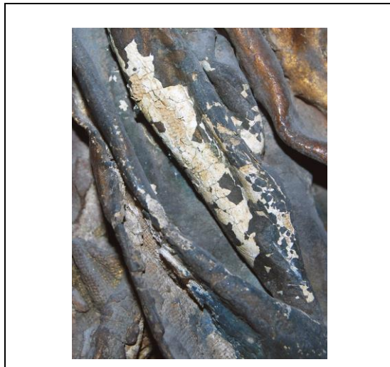
Figure 2. Deadhesion and decohesion defects.
